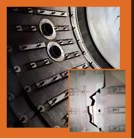
It is no surprise that equipment located near the turbine exhaust typically demands more frequent maintenance and repairs. The high operating temperatures up to 1200°F and gas flow causes wear on the material creating overheating issues that could lead to premature equipment failures or exhaust leaks. The A042 transition diffuser duct is an area that is typically exposed to these leaks and potential damage.
